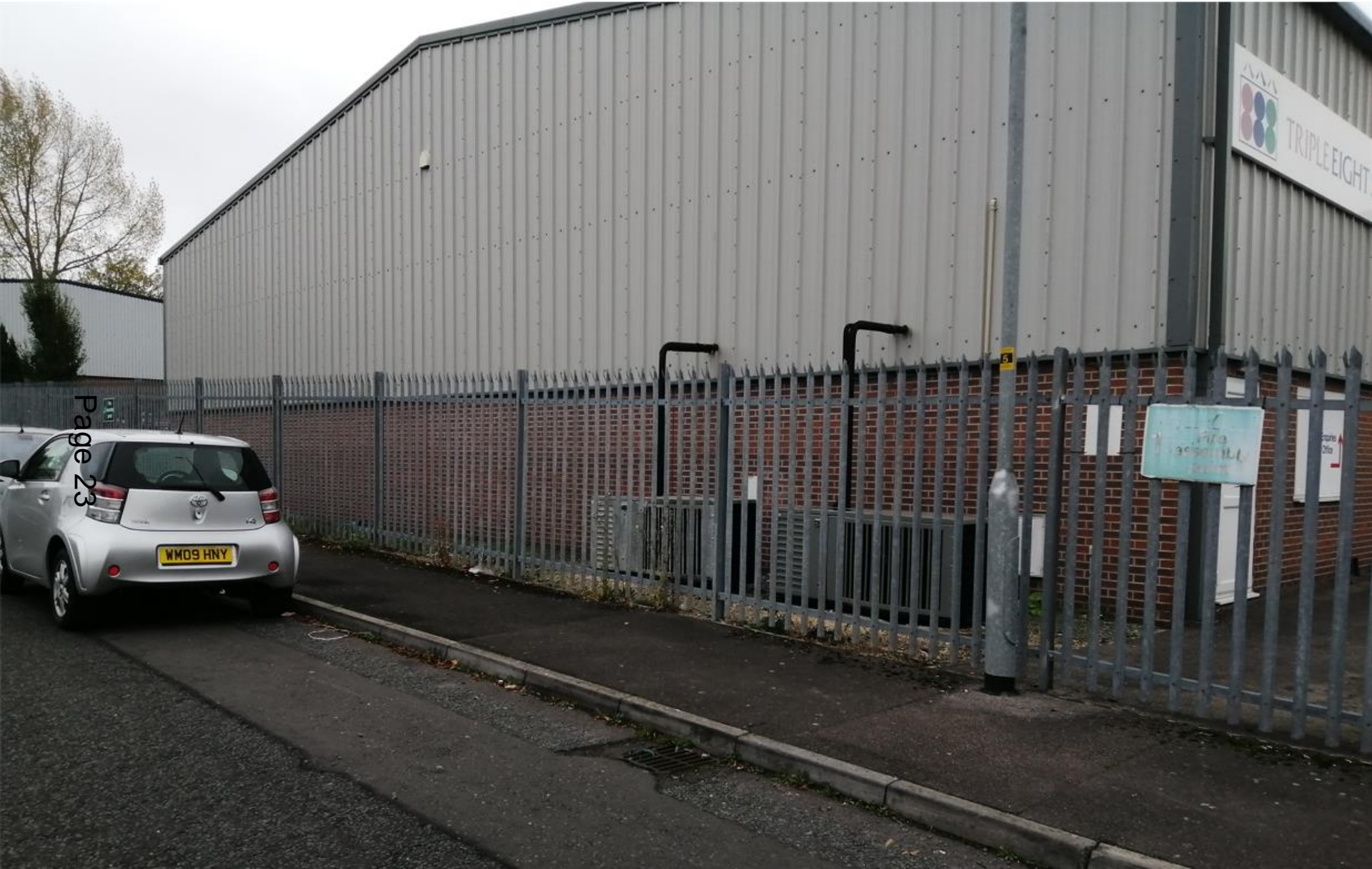
Photograph of Triple Eight Supplies unit opposite the application site
