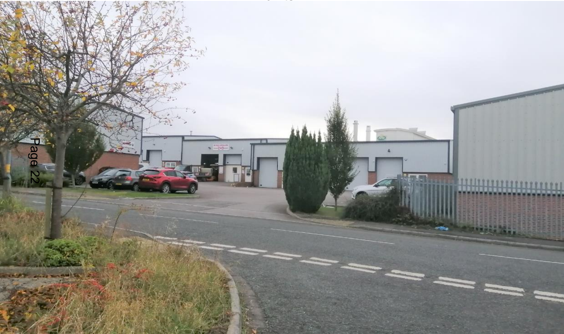
Photo of the 'Curtis Centre' from the junction to the Sorting Office – comprising of 13 units
